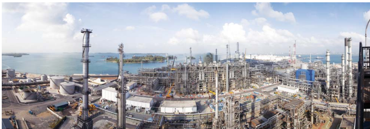
The ethylene cracker at Shell Eastern Petrochemical Complex in Singapore.
